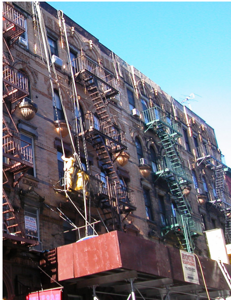
Lower East Side tenement buildings
